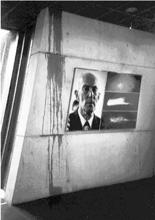
Figure 8. My installation in the entry hall of the J.H. Oort Building in Leiden, showing a portrait of Jan Oort at 80 years, flanked by images of the Crab Nebula, Comet Halley, and a hydrogen channel map of the Milky Way. The streaks on the left are water damage due to construction flaws in the new building.
